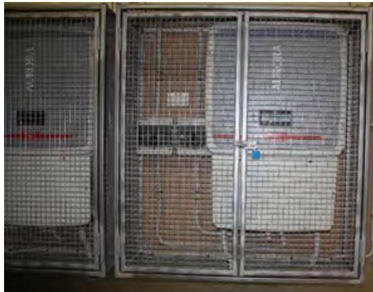
Fig. 9.2.3 Access to inverter is controlled
