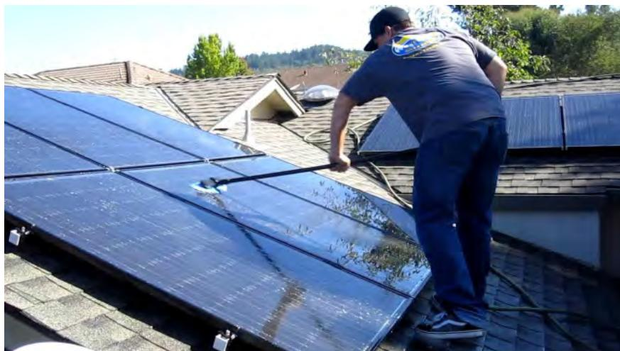
Fig. 10.2.2 Cleaning modules using a mop
