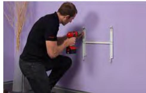
Fig. 8.2.6 Installation of Inverter mounting structure
