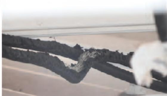
Fig. 9.3.3 Poor quality conduit and unprotected cable can be easily damaged
