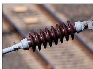
Fig 2.2.11 Insulator – ceramic
