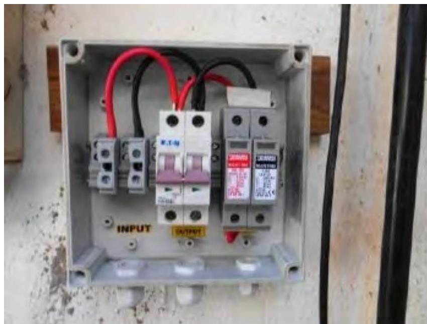
Fig. 8.3.6 AC distribution box (AC MCB for AC isolation, Surge protection device and Input side fuse protection)
