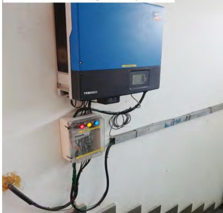
Fig. 8.5.7 Inverter and AC distribution box
