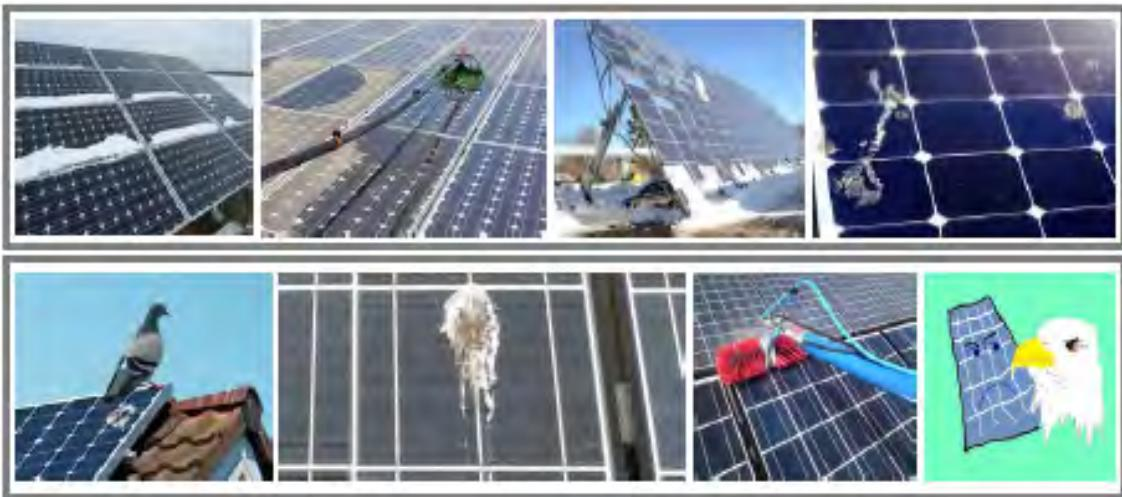
Fig. 12.1.2 Clean without stepping on the panels or placing heavy objects on them
