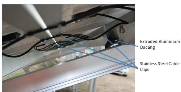
Fig. 9.3.2 Properly managed PV array cable
