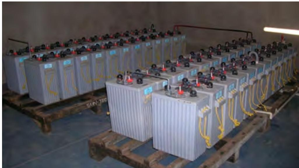
Fig. 9.2.5 Location of batteries in a well ventilated room
