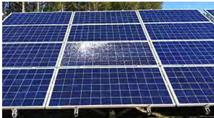
Fig. 10.2.3 Broken module in a PV array
