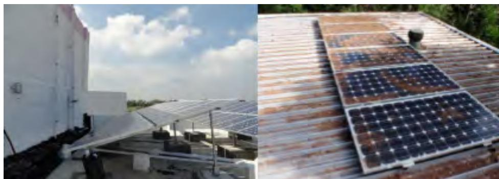
Fig. 9.2.2 Incorrect site selection for array installation
