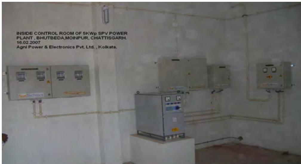
Fig. 9.2.4 Inverter and control equipment installed in a control room
