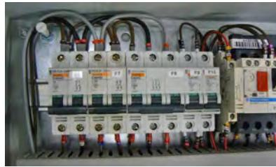
Fig. 5.2.3 Miniature Circuit Board (MCB)
