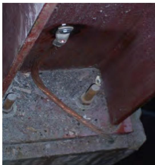
Fig. 8.4.1 Connection of ground wire to metallic part of a building
