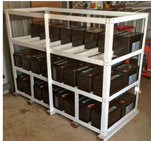
Fig. 8.5.1 Battery Bank enclosures/racks
