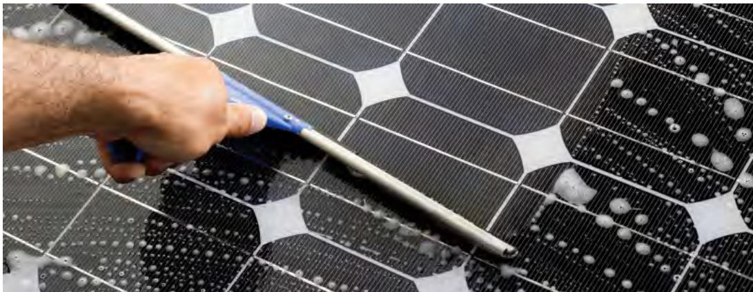
Fig. 10.2.1 Cleaning of modules using a wiper
