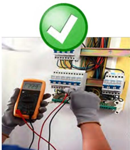
Fig. 11.2.5 Right way: Use protective hand gloves
